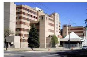
the vacant building
